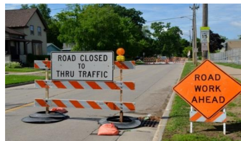
Figure 3: Road Work Ahead & Temporary Barricades
