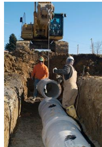
Figure 2a: Installation of drainage
